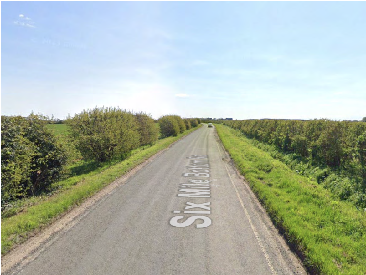
Figure T&T 2a Six Mile Bottom Road is a narrow double track road with soft verges, deep drainage ditches and few passing places.
